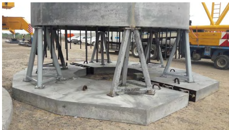
Fig. 29 Concrete slab for tower sections preassembly – concrete tower.
