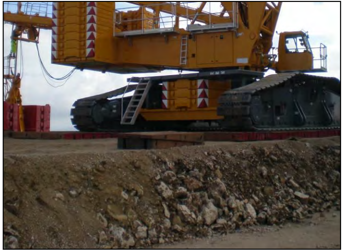
Fig. 27 Wooden sleepers under the crane to prevent excessive ground deformations.
