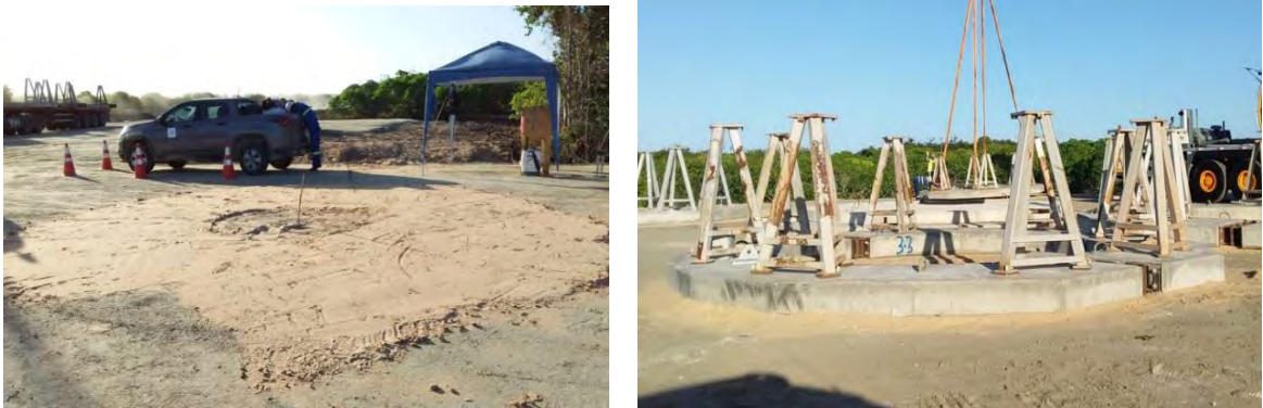
Fig. 30 Concrete slab onto layer of sand.
