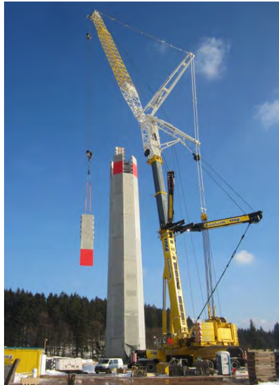
Fig.10 TCS164NV05 and TCS164NV06 type concrete tower keystone erection.
