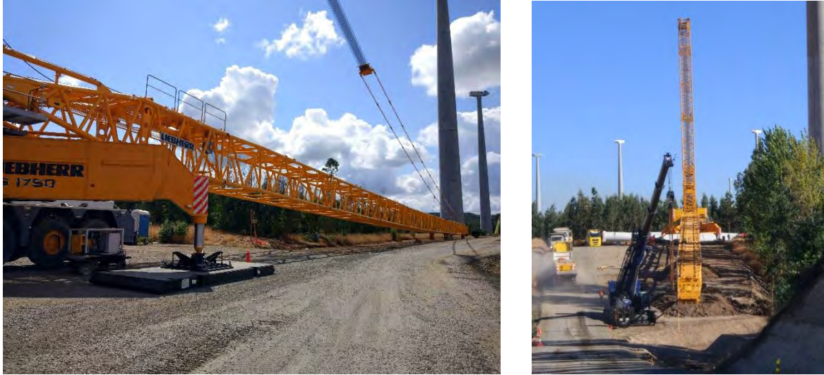
Fig. 28 Crane boom assembly area example.
