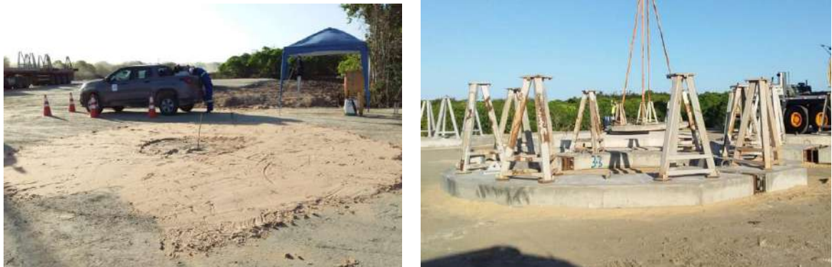
Fig. 30 Concrete slab onto layer of sand.
