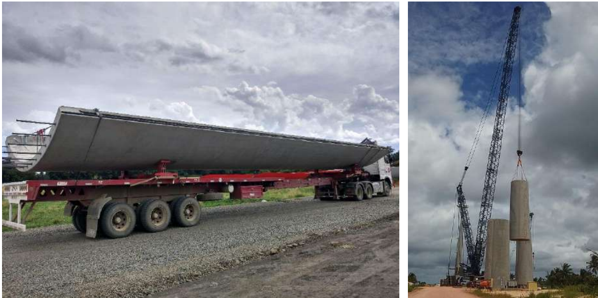
Fig.8 Transportation of a TC120N and TCS164N type keystone.
