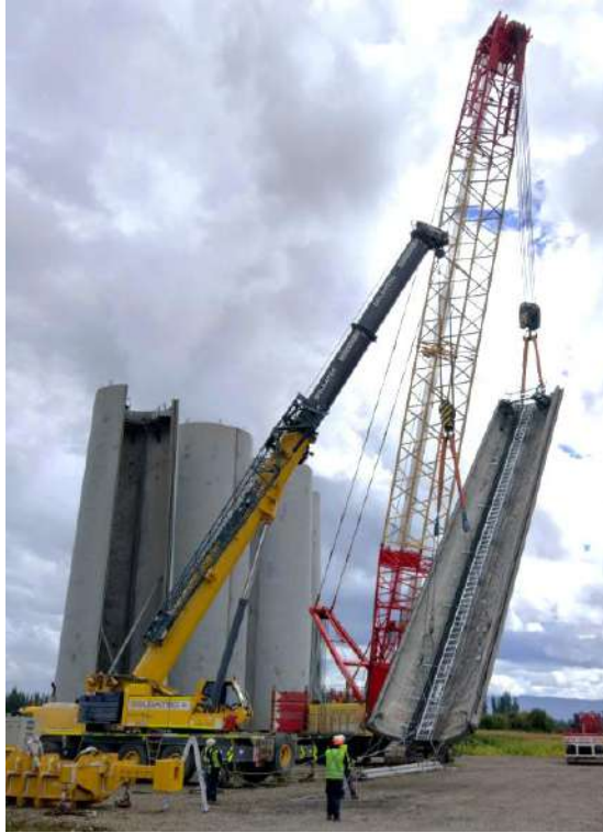
Fig.9 TC120N and TCS164N type concrete tower sections' preassembly.
